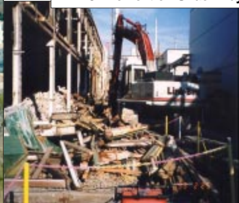
K-1131 Demolition Under Way
